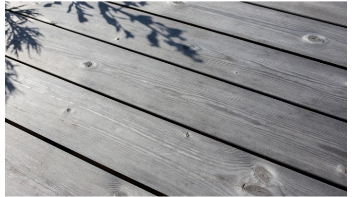
Thermory Benchmark thermo-pine decking, aged and unoiled.
